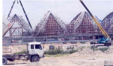
New International Airport under construction
